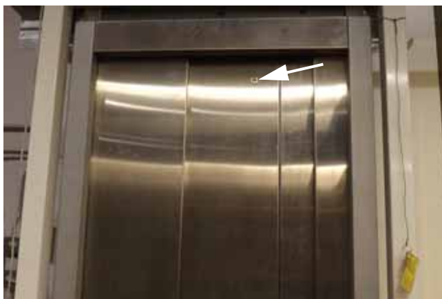
Figure 4: Auto Slim Landing Doors Emergency Opening
